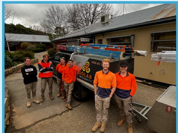
TRY Grant – Solar Integrity installing Solar and Battery on YCC.
